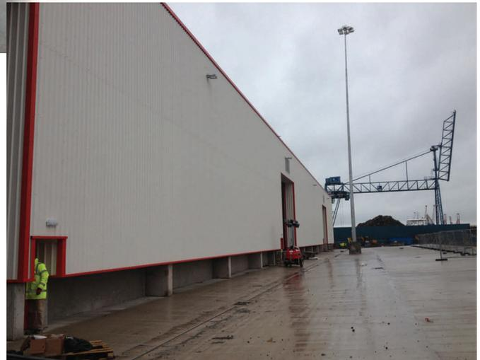
Following extensive consultations internally at Bristol, with Forth Ports and with the main contractor, the Bristol Port management ordered the Dialight 17,000 lumen, 172W LED High Bay fittings. These were installed along with the latest LED 126lm/W floodlights which were located on the external walls of the biomass storage facility. Both LED luminaires come with a 10 year full performance warranty from a UK plc.
